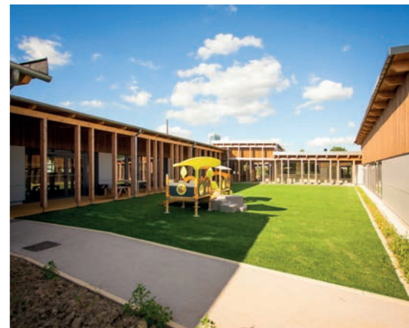
photos service communication Verdun/Garonne
